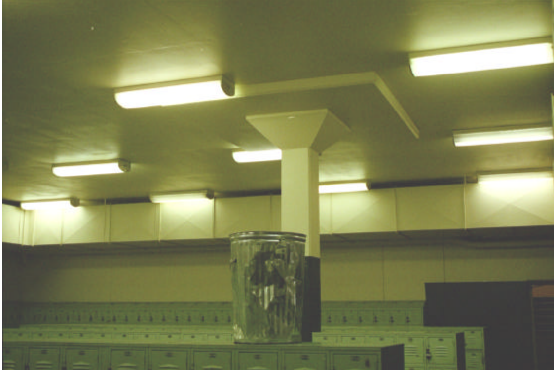
Figure 16: Gymnasium Building (Unit 6), interior locker room
