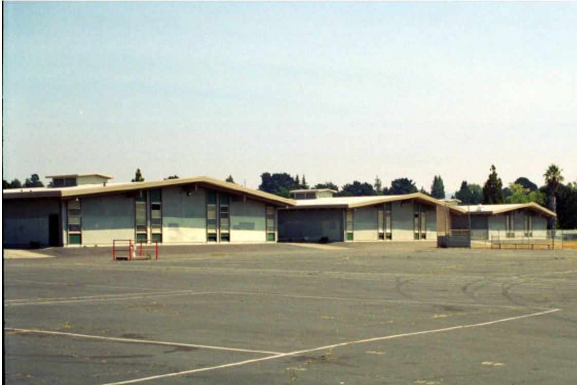
Figure 4: Classroom Buildings (Units 1, 2, & 3), exterior west wall
