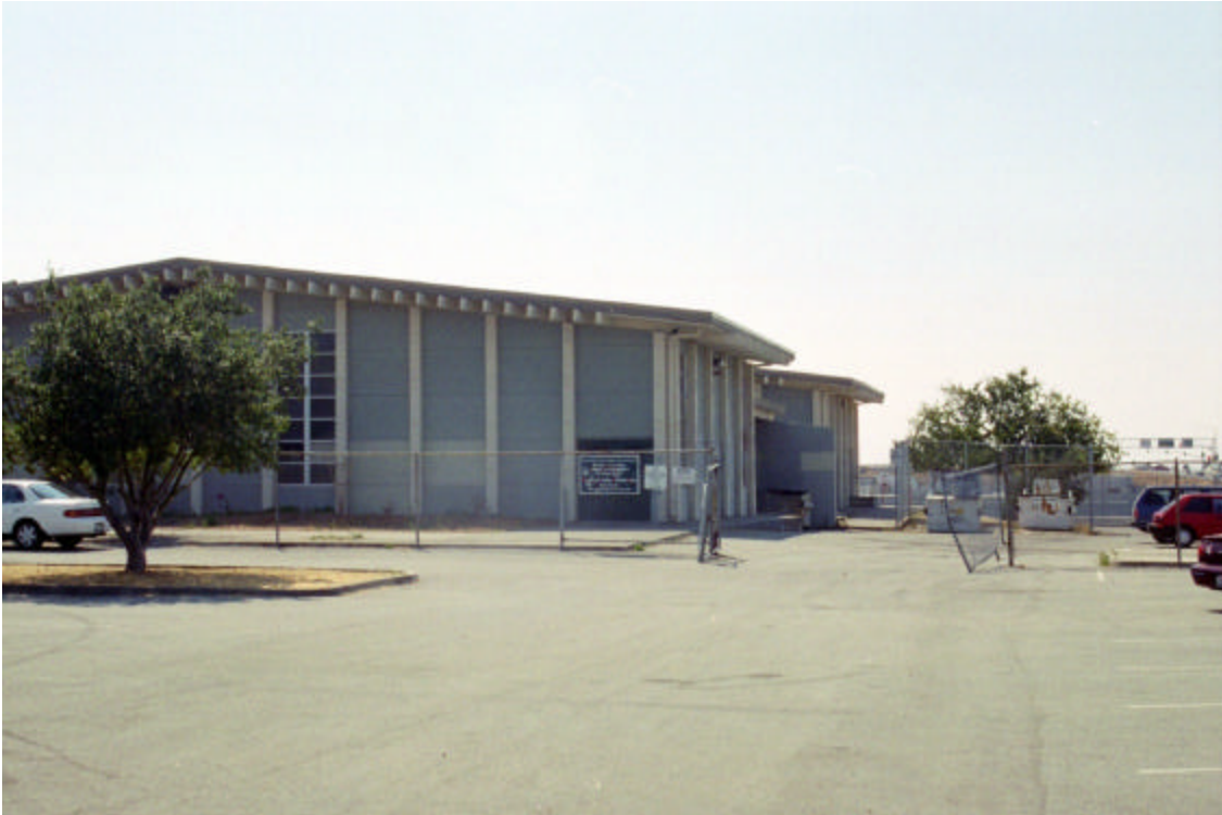
Figure 11: Cafeteria/music Building (Unit 5), exterior northeast corner
