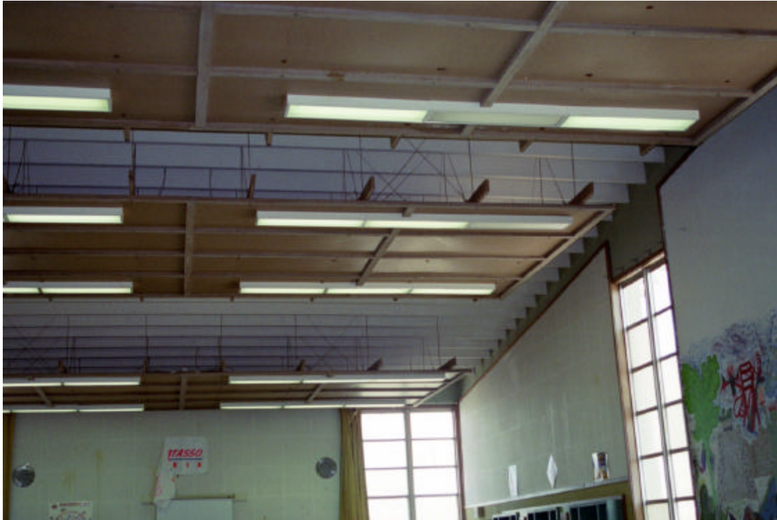
Figure 12: Cafeteria/music Building (Unit 5), interior ceiling
