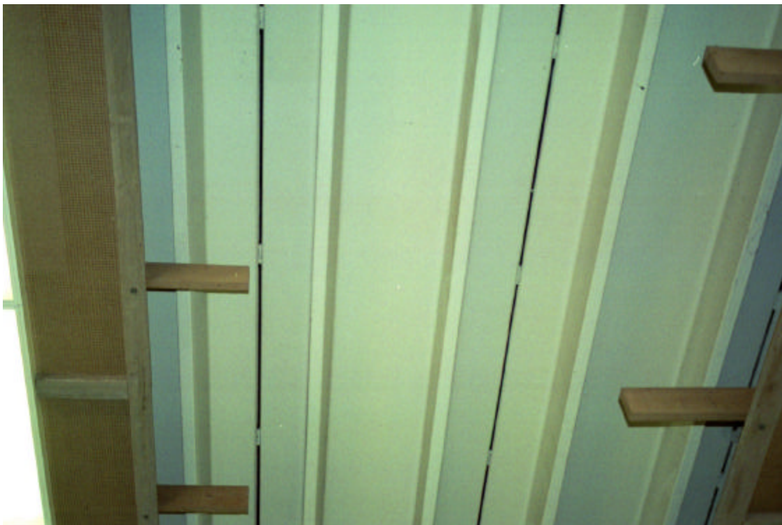
Figure 13: Cafeteria/music Building (Unit 5), interior pre-cast joist flange splice
