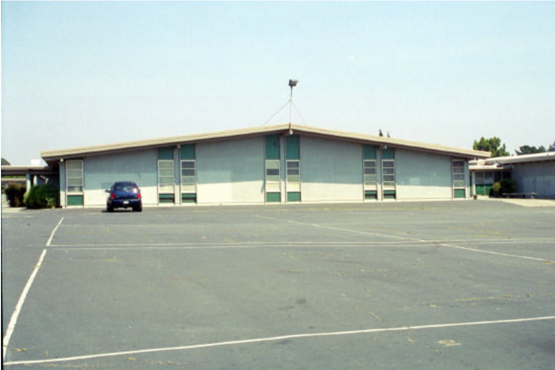
Figure 3: Library/administration Building (Unit 4), exterior west wall
