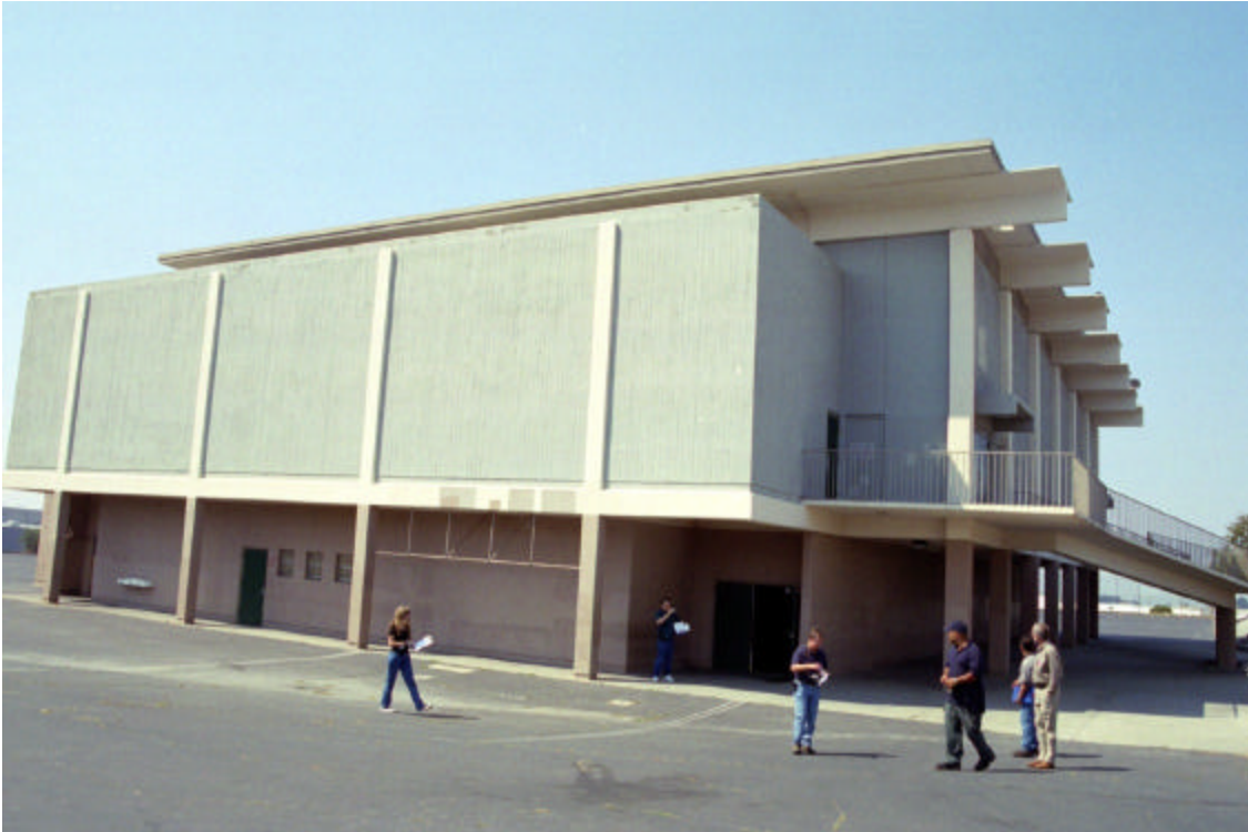
Figure 15: Gymnasium Building (Unit 6), exterior southeast corner
