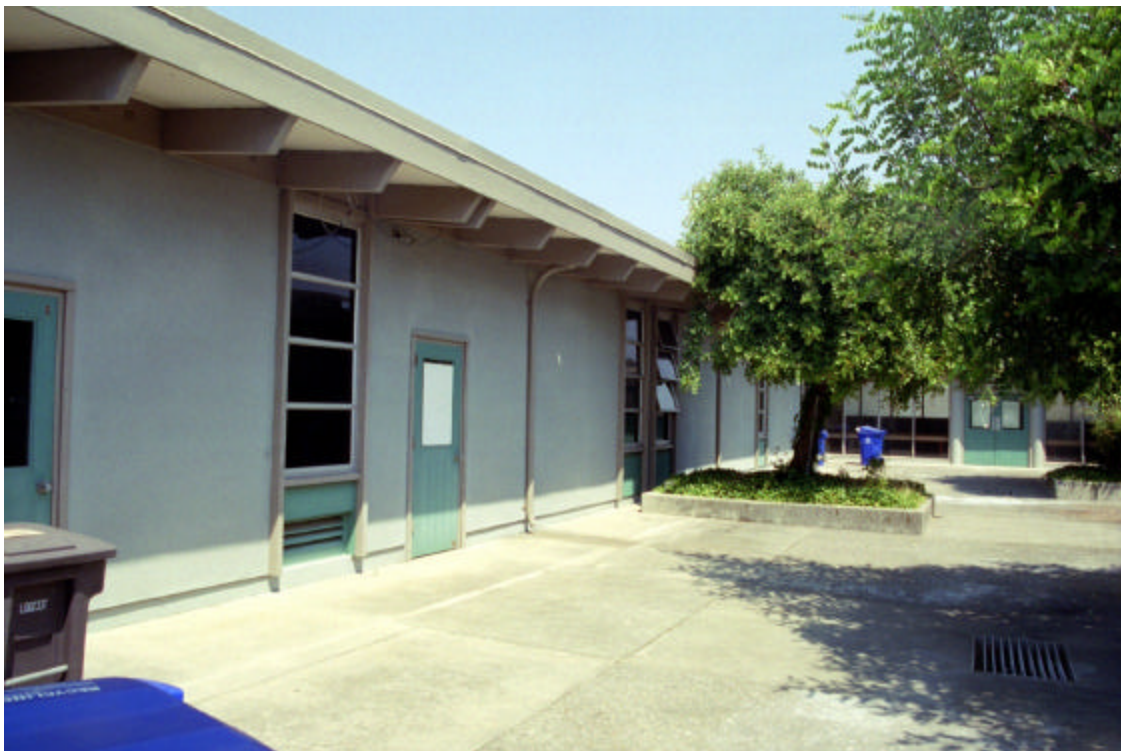
Figure 7: Typical Classroom Building (Unit 1, 2, 3, 4, 8), exterior longitudinal wall
