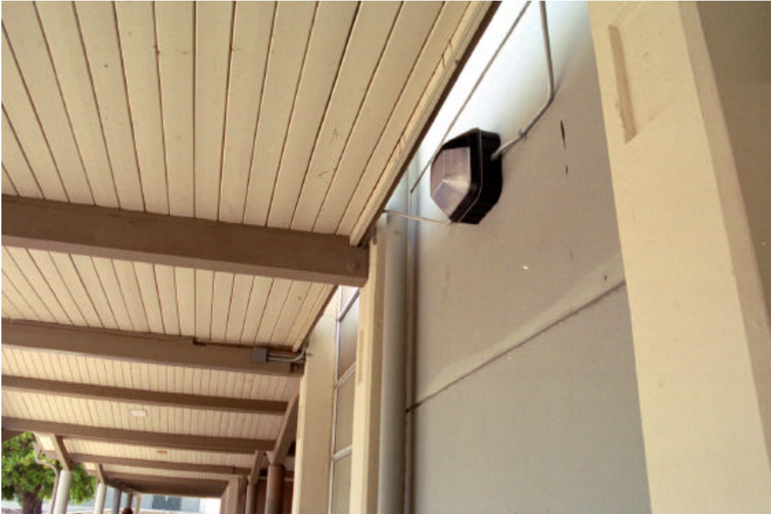
Figure 19: Covered Walkway, hard conduit
