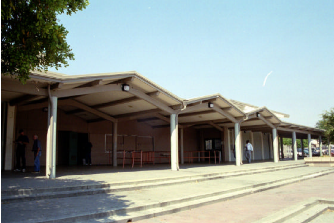
Figure 10: Cafeteria/music Building (Unit 5), exterior south covered walkway
