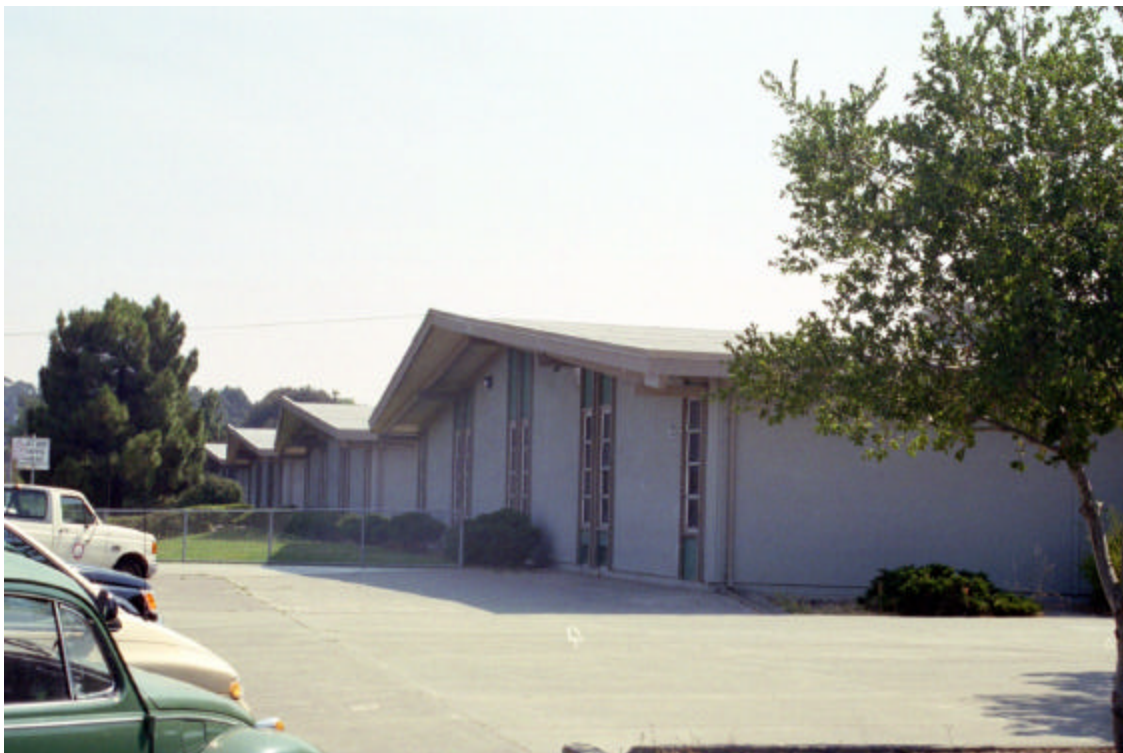
Figure 5: Classroom Buildings (Units 1, 2, 3 & 4), exterior east wall
