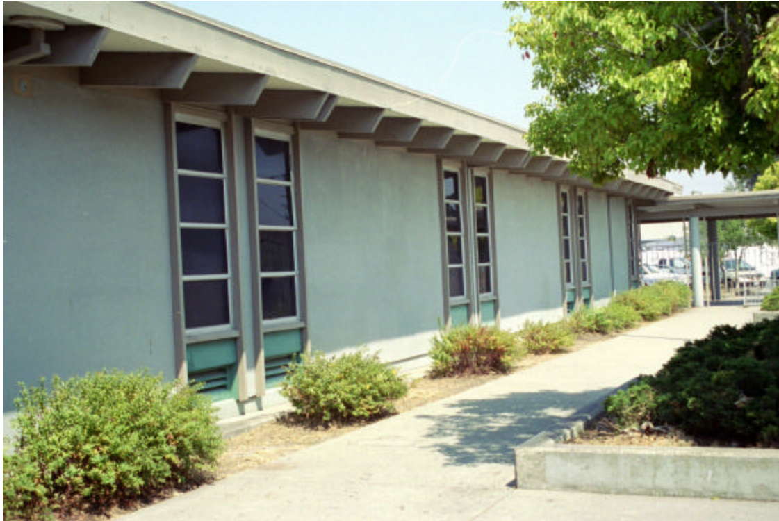
Figure 6: Typical Classroom Building (Unit 1, 2, 3, 4, 8), exterior longitudinal wall
