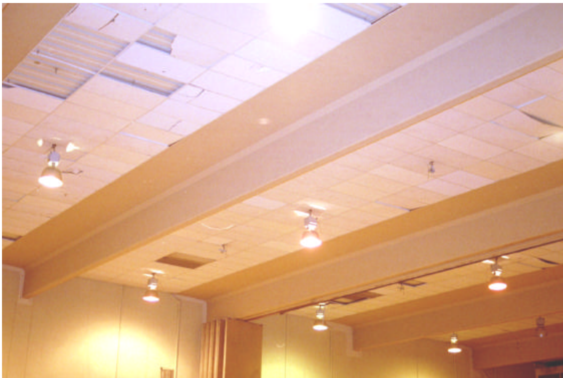
Figure 17: Gymnasium Building (Unit 6), interior gymnasium
